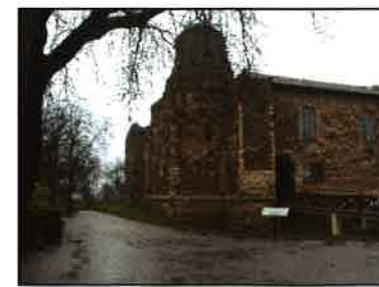
Photo 7 Castle Museum entrance bridge.
