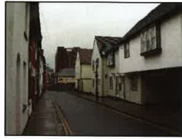
Photo 56 Looking up West Stockwell Street northwards to Northgate Street.
