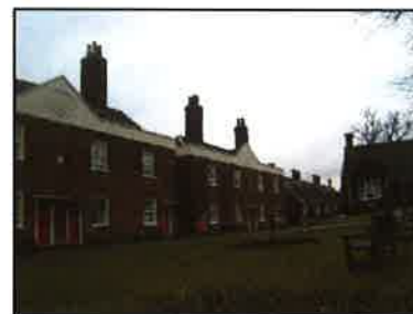
Photo 119 Historic Kendalls Almshouses.
