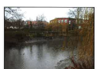
Photo 73 Middle Mill on River Colne - looking south towards Town Centre.
