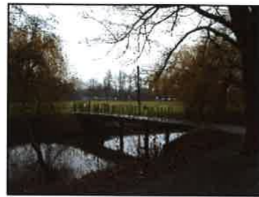
Photo 74 Footbridge across to Cricket Ground from Lower Castle Park.
