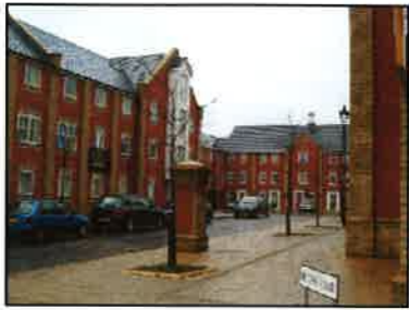
Photo 101 New Housing at Hesper Road off Hythe Quay.
