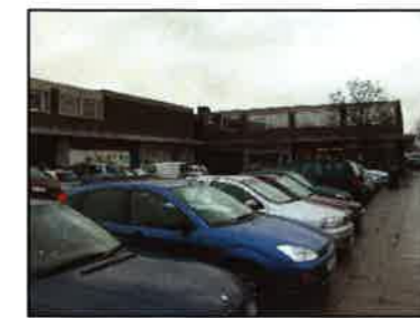
Photo 138 Old shopping centre, corner of Church Street/New Road.
