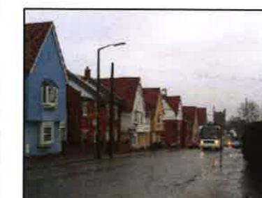
Photo 90 New housing at Edward Paxman Gardens, off Hythe Hill.
