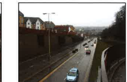
Photo 46 Balkerne Hill looking north from Footbridge.
