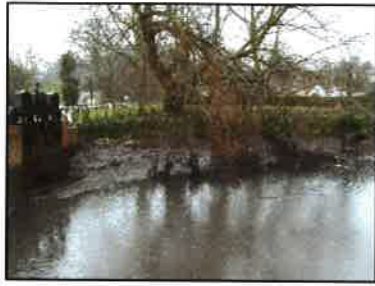
Photo 73 Middle Mill on River Colne - looking south towards town centre.
