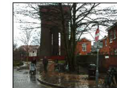
Photo 45 Mercury Theatre - Jumbo water tower.
