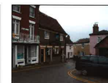
Photo 192 Black Buoy Hill from East Street.
